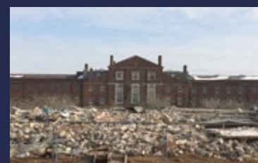
Cross Link demolition 2018
